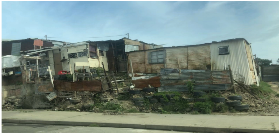
Figure 7. Housing modification applied by residents over time
