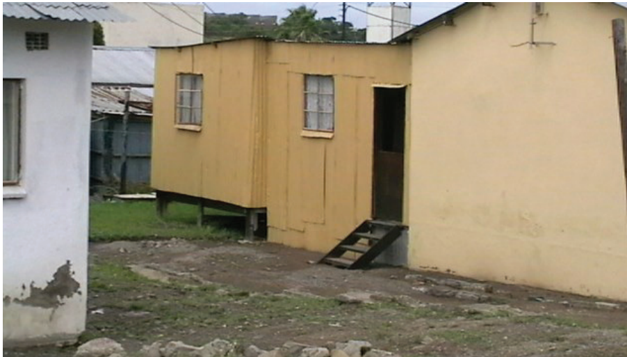
Figure 8. Raised housing modification to prevent flooding of structure
